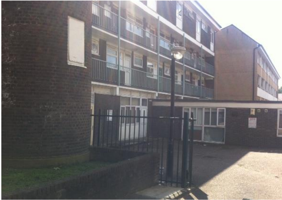
Photo 3: Rear of the building
