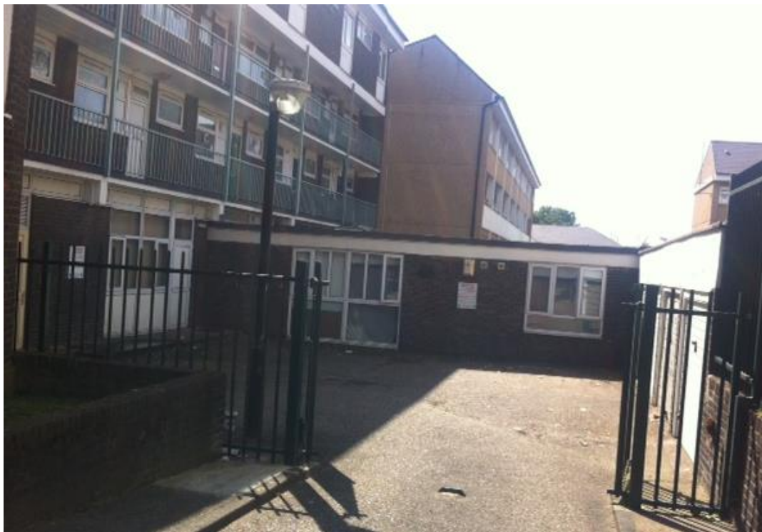
Photo 4: Rear of building
